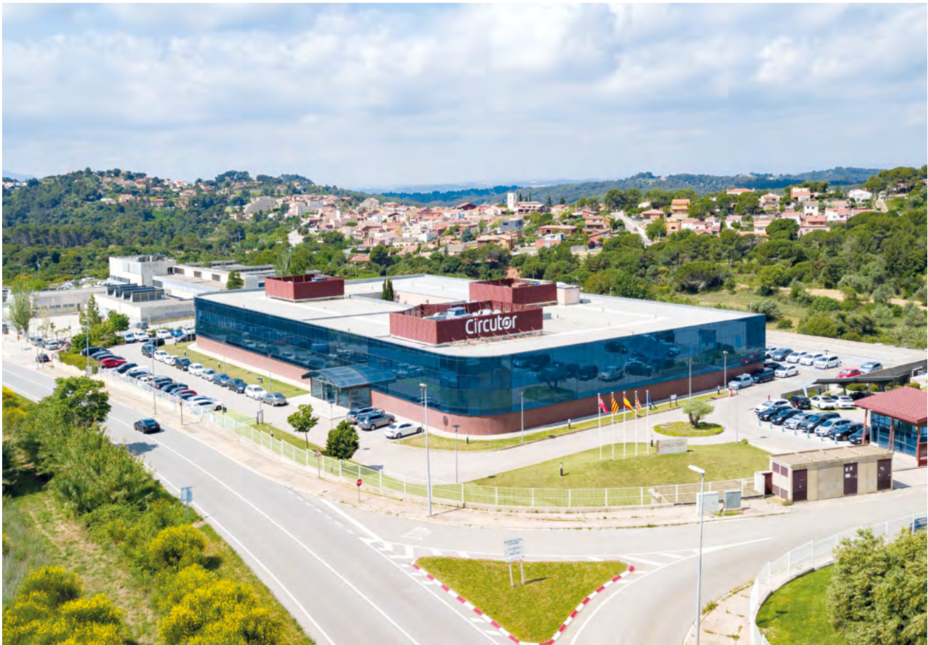
CIRCUITOR headquarters in Viladecavalls, Barcelona.
